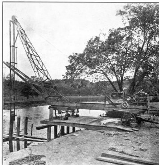
PILE DRIVING FOR FOOTBRIDGE BY ENGINEERS IN FRANCE.
