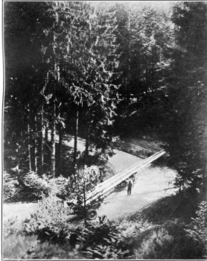
TRUCKS LOADED WITH PILING EN ROUTE TO FRENCH RAILWAY YARDS NEAR BRUYERS, FRANCE.
