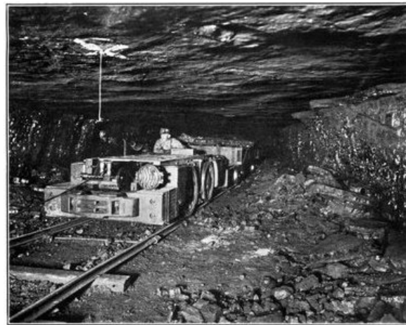
6-TON ELECTRIC LOCOMOTIVE PULLING A STRING OF COAL CARS.
