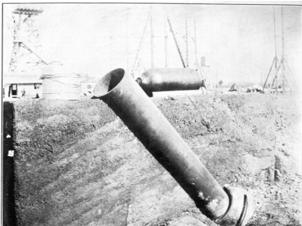
EIGHT-INCH LIVENS PROJECTOR, MARK II, WITH POWDER CHARGE AND SHELL.
