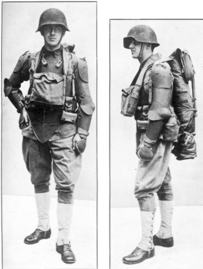
AMERICAN EXPERIMENTAL MODELS OF HELMETS, LIGHT BREASTPLATES, AND ARM GUARDS.
