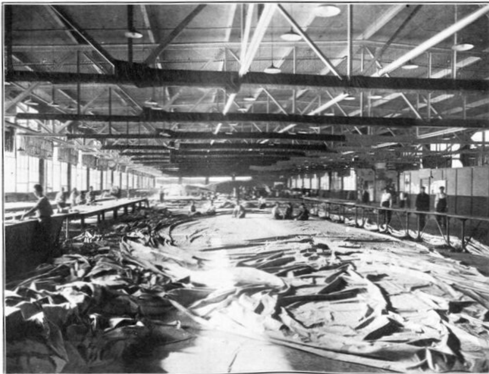
FINAL BALLOON ASSEMBLY ROOM AT GOODRICH FACTORY.
