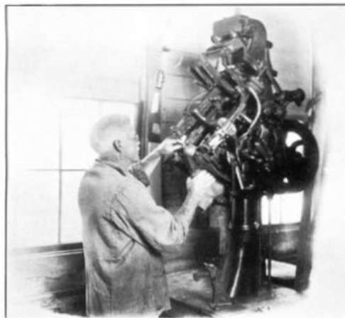
Pulling Upper Over Last. MANUFACTURING ARMY SHOES.
