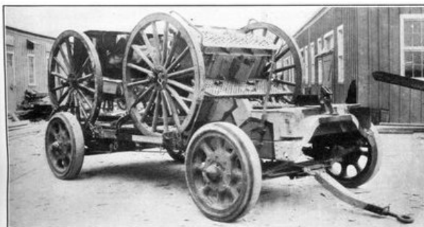
THREE-INCH FIELD GUN TRAILER. A specially designed vehicle for carrying different loads, including a 3-inch field-gun carriage and limber in one load and two 3-inch field-gun caissons for another load.
