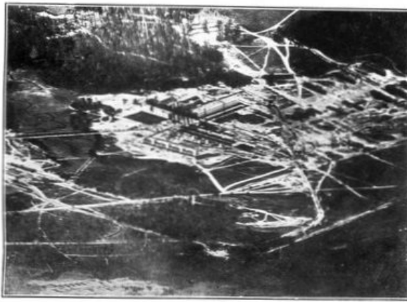
AIRPLANE VIEW OF CHLORINE PLANT, EDGEWOOD ARSENAL.
