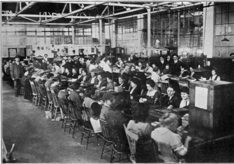
MARK V FUSE ASSEMBLY.
