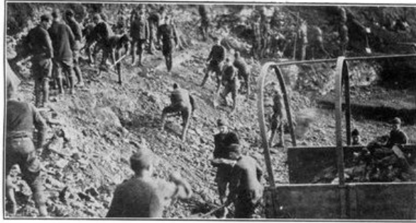
AMERICAN ENGINEERS QUARRYING STONE TO REPAIR MILITARY ROADS DESTROYED BY GERMAN SHELL NEAR MENIL-LA-TOUR, FRANCE.
