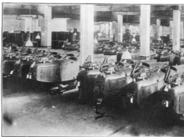
HALL-SCOTT ENGINES BEING INSTALLED IN AIRPLANE FUSELAGES.
