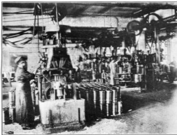
DRILLING CYLINDER FLANGES WITH MULTIPLE DRILL. PACKARD MOTOR CAR CO.
