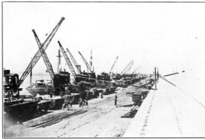
NORTHERN VIEW OF THE AMERICAN DOCKS AT OLD BASSENS, BORDEAUX, FRANCE.
