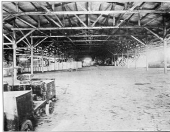
INTERIOR VIEW OF ONE OF THE LARGE WAREHOUSES AT BASSENS DOCKS, BORDEAUX, FRANCE.
