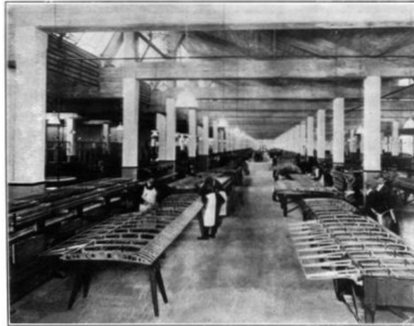
ASSEMBLING DE HAVILAND-4 WINGS AT THE DAYTON-WRIGHT PLANT.
