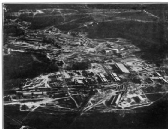
IN THE FOREGROUND THE CHLORINE PIPE LINE FROM CHLORINE PLANT
