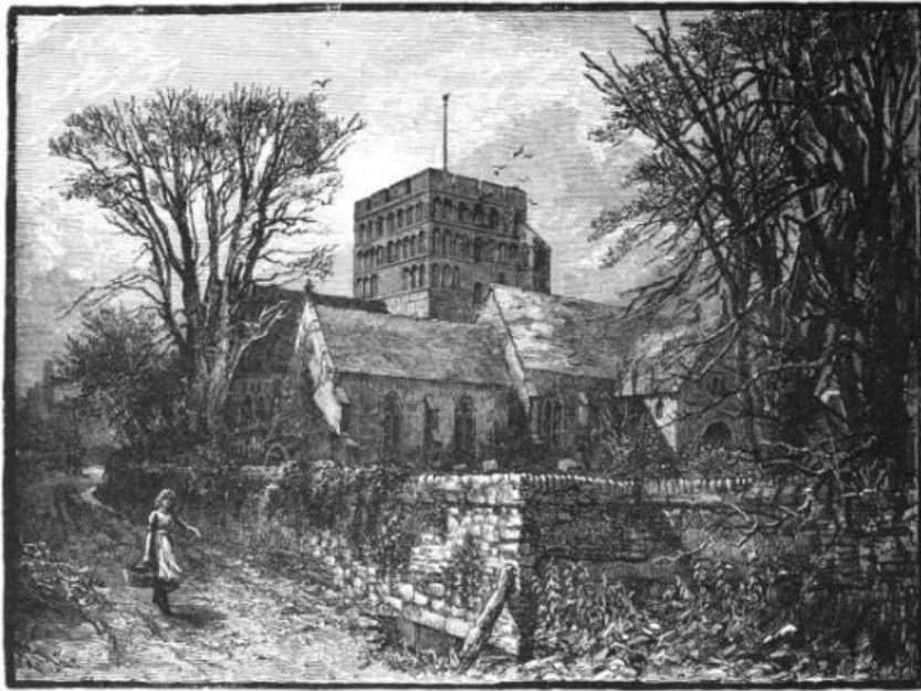
ST. CLEMENT'S, SANDWICH, SHOWING THE NORMAN TOWER.
