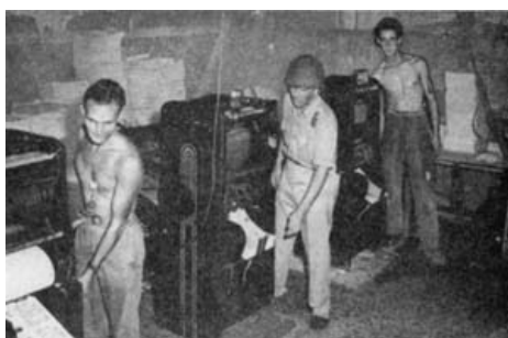
Figure 39: Leaflet Production: Military Presses. The machines shown are Davidson presses, widely used by the Americans in all theaters of war. The unit shown is Psychological Warfare Branch during the Leyte operations. The leaflet being run off is addressed to both Filipino guerrillas and Japanese troops, facilitating a difficult three-way operations whereby Japanese are told to surrender to Filipinos, Filipinos told not to kill surrendering Japanese, and Americans instructed to receive prisoners from Filipinos.
