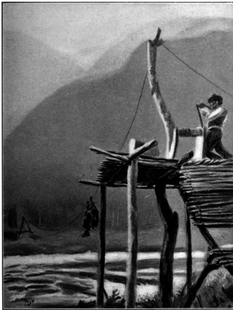
On the Rope a Trolley Worked Back and Forth from which was Suspended a Tiny Platform
