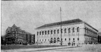
PIERCE BUILDING PUBLIC LIBRARY
