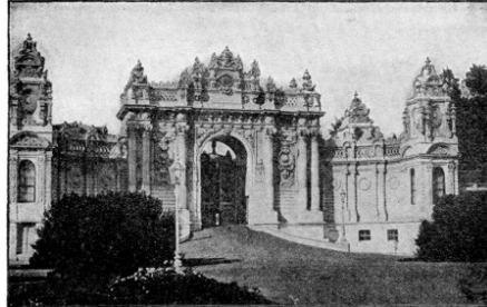
ENTRANCE TO DOLMA-BAGTÇHE PALACE
