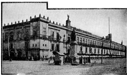
NATIONAL PALACE, CITY OF MEXICO
