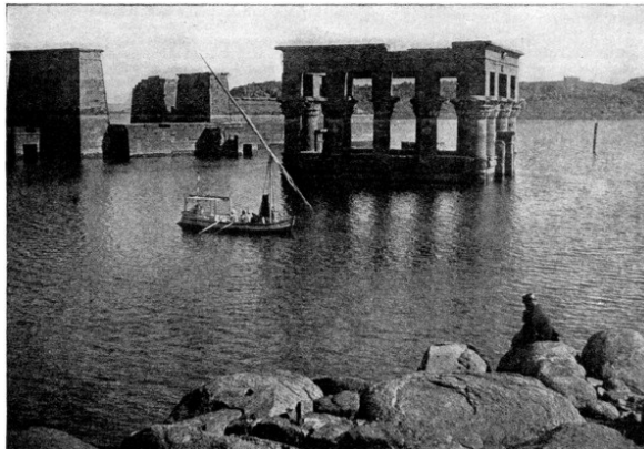
This is a view of the great dam at Assuan, across the Nile in upper Egypt, showing the ruins of the beautiful Temple of Philæ partially submerged. The Assuan dam was the largest in the world until the completion of the Elephant Butte dam, New Mexico, in May, 1916.
