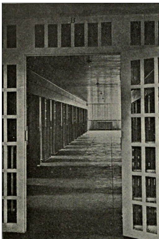
CELL BLOCK CORRIDOR
