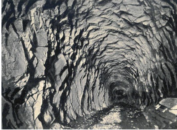
Summit tunnel (altitude 7,042 feet) before completion—Sierra Nevada Mountains
