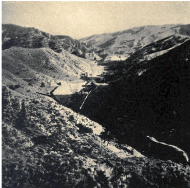
View south from over the San Fernando tunnel—Southern Pacific Railroad
