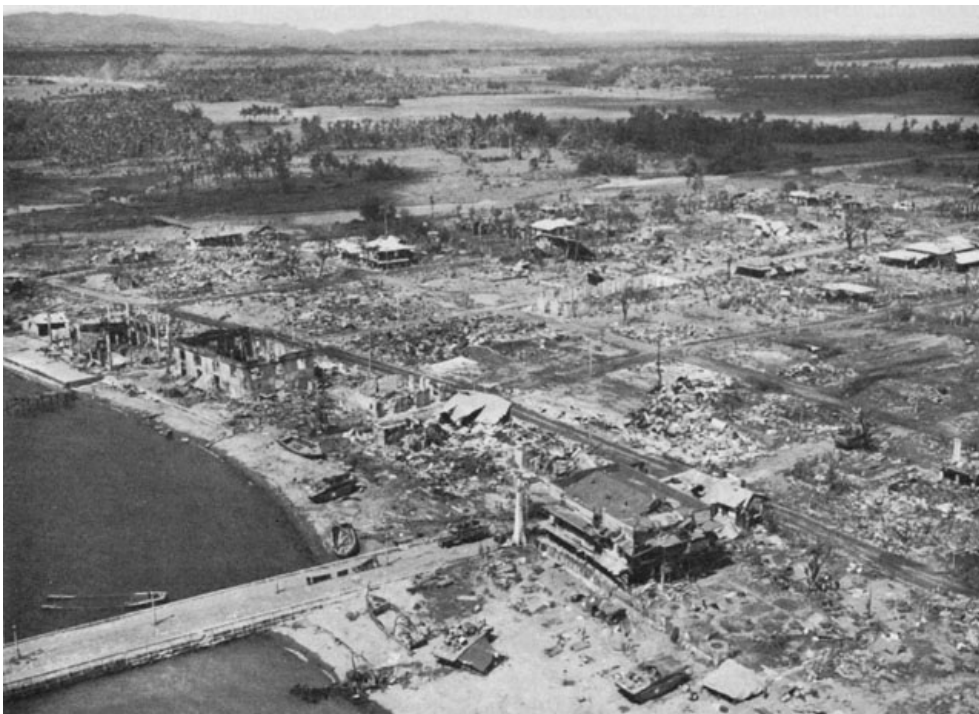
AERIAL VIEW OF ORMOC after the bombardment. In the middle background is the Antilao River, with the mountains of western Ormoc Valley in the distance.
