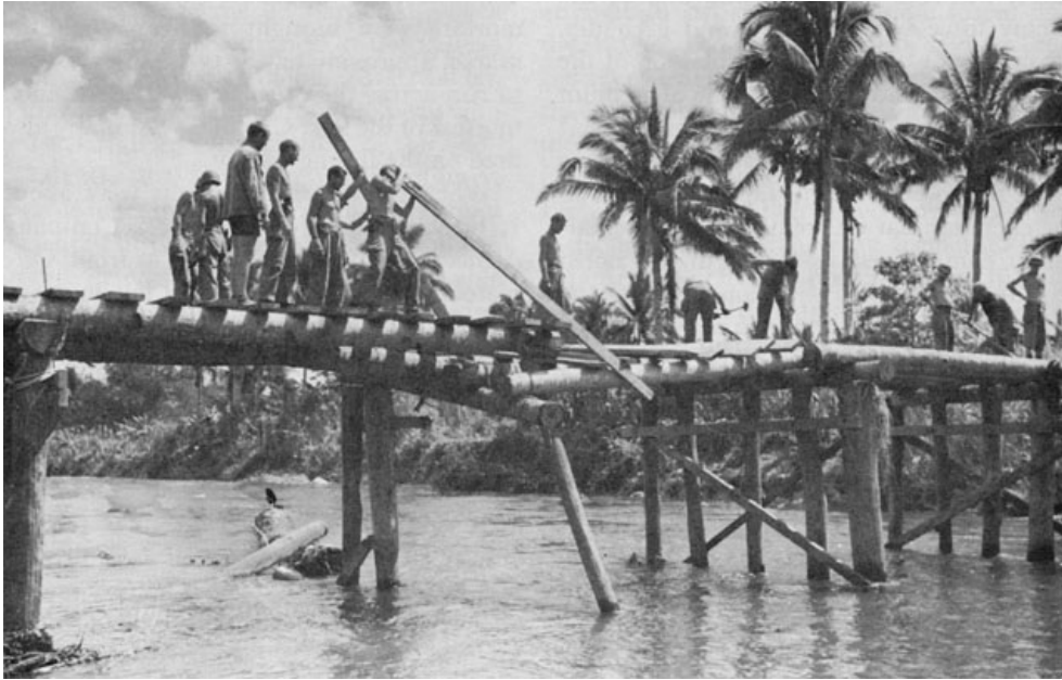
ENGINEER TROOPS of the 13th Engineer Battalion rebuild a bridge near Burauen.
