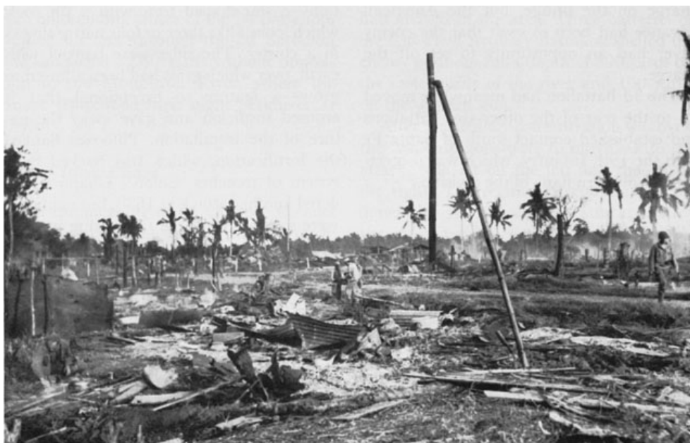
PASTRANA was left a mass of smoldering ruins after the shelling of 26-27 October.
