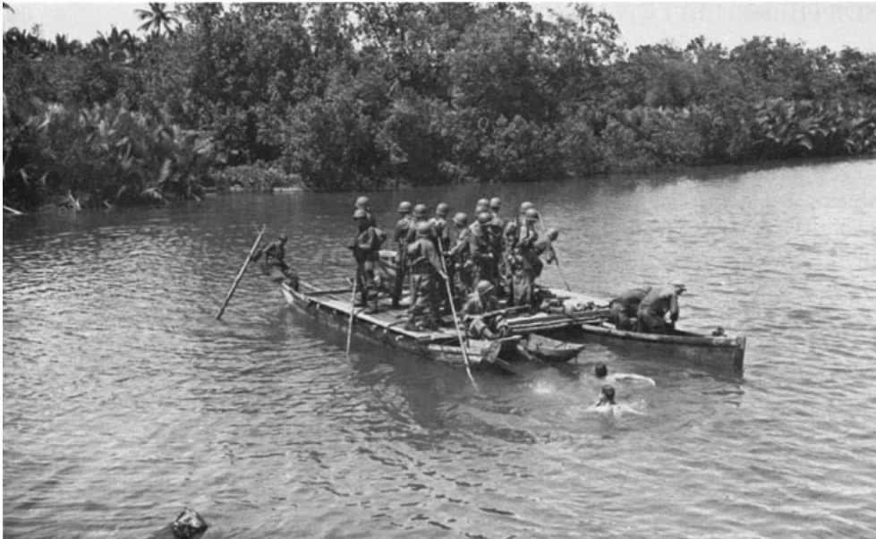
U.S. PATROL CROSSING THE CANOMONTAG RIVER (above). Engineer troops replacing a Capoocan River bridge blown up by retreating Japanese.
