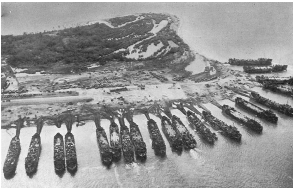
LST'S UNLOADING AT TACLOBAN AIRFIELD. The causeways leading from the beach to the ships were built by bulldozers scraping sand and earth to each ship as it landed.
