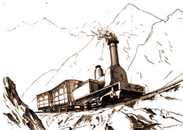
A CENTRE RAIL ENGINE AND TRAIN ASCENDING A GRADIENT OF 440 PER MILE WITH A CURVE OF 44 YARDS.
