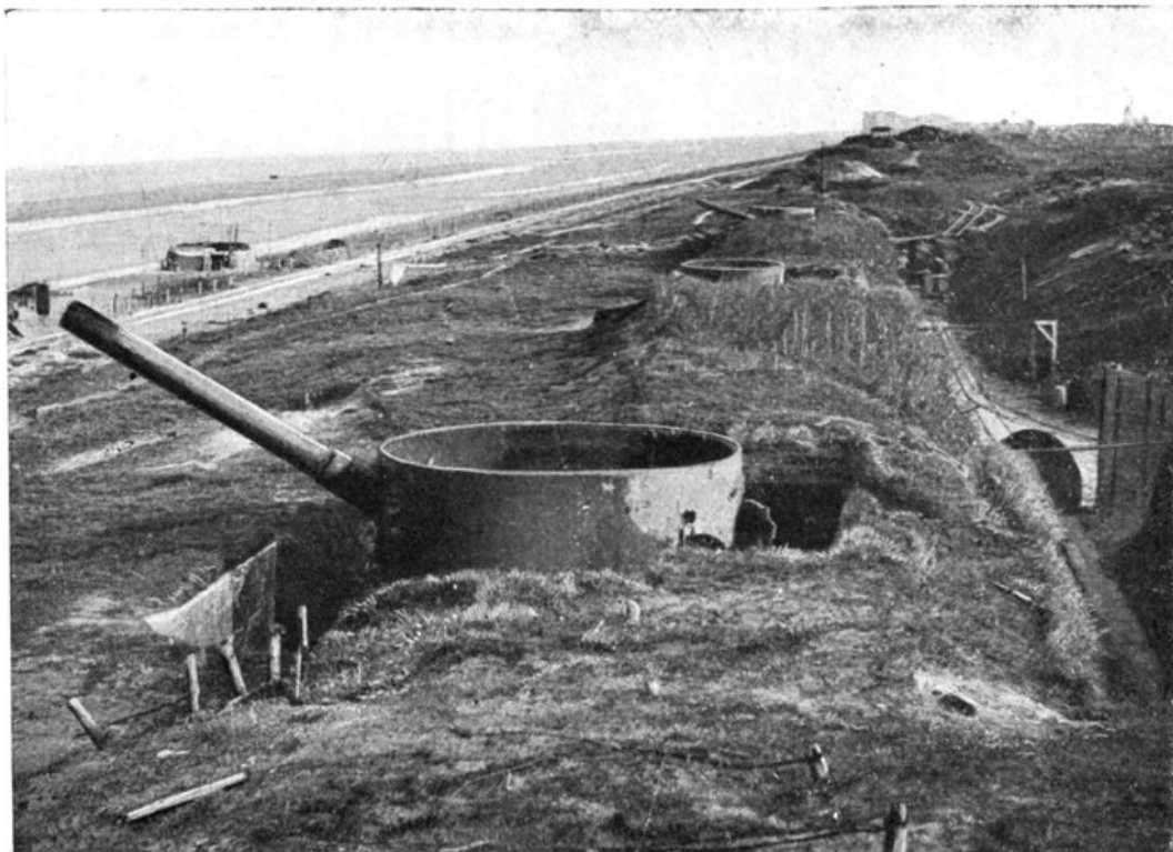
GENERAL VIEW OF THE AACHEN BATTERY (north-east of Middelkerke-Bains.)
