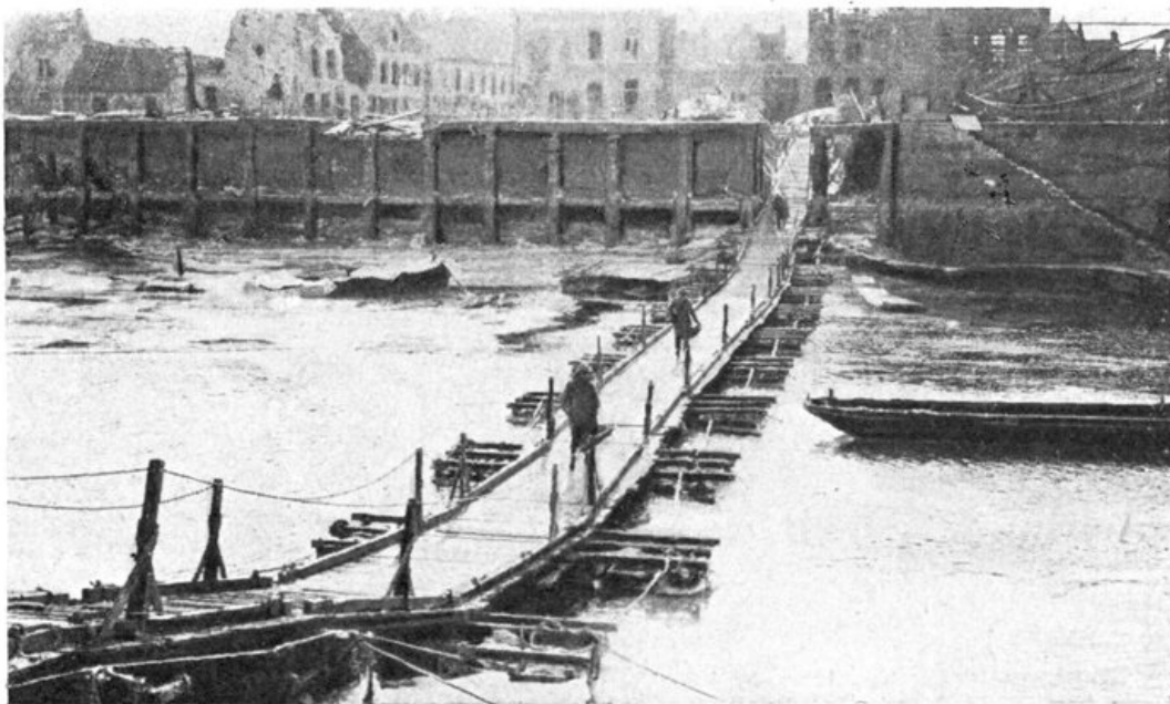
TEMPORARY FOOT-BRIDGE ACROSS THE YSER AT NIEUPOORT.
