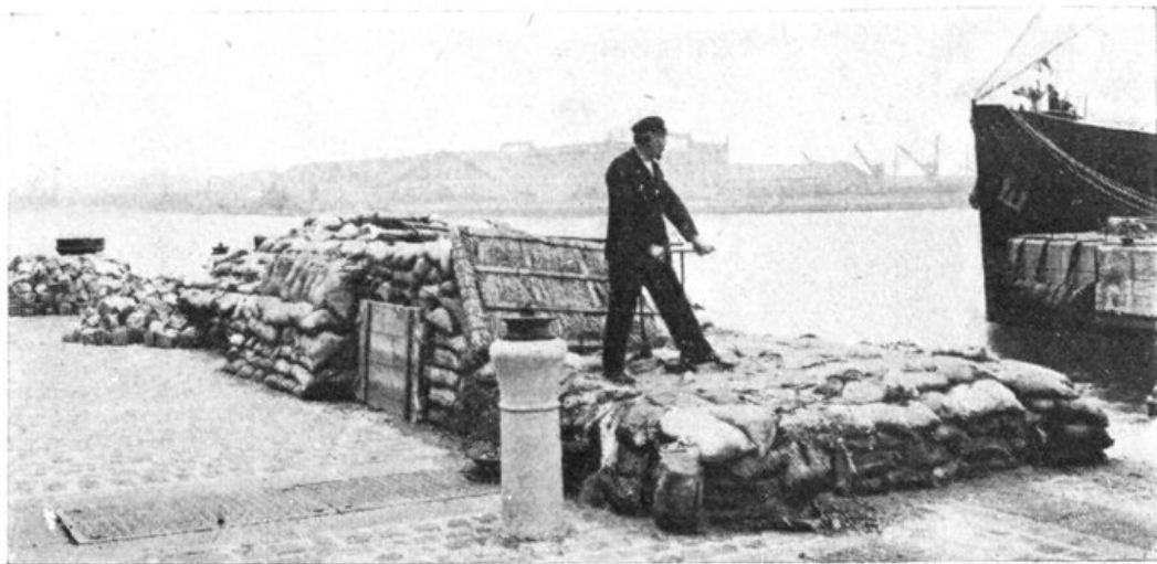
PROTECTING THE MECHANISM OF THE LOCKS FROM THE SHELLS.
