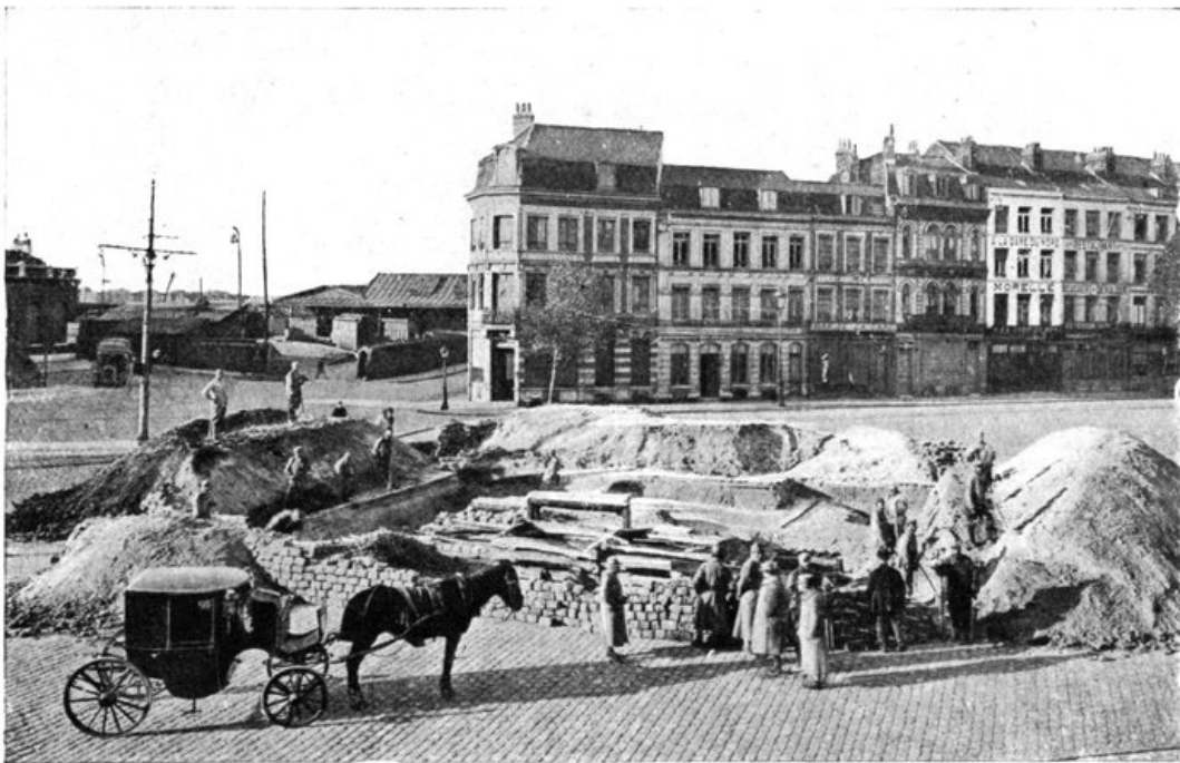
BUILDING A BOMB-PROOF SHELTER IN FRONT OF THE STATION.
