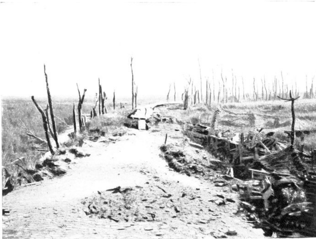
TEMPORARY BRIDGE AT TERVAETE, ON THE IMPASSABLE ROAD TO STUYVEKENSKERKE, IN 1919.
