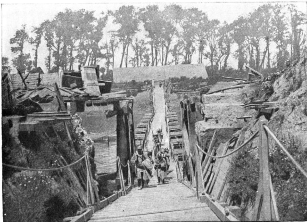
PONTOON BRIDGE ACROSS THE YSER.
