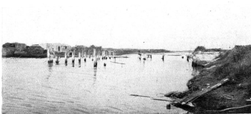
THE PONT DE L'UNION, BETWEEN ST. GEORGES AND MANNEKENSVERE.
