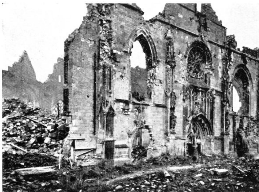
THE FAÇADE OF ST. JEAN CHURCH IN 1919.
