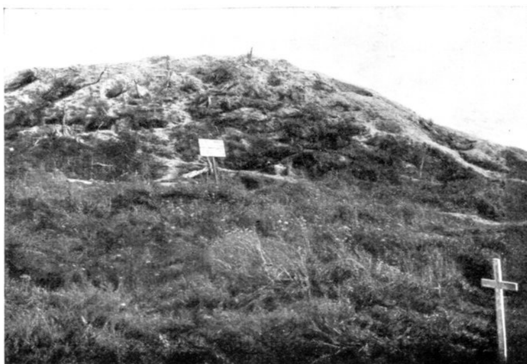
ENTRANCE TO THE UNDERGROUND DEFENCES.
