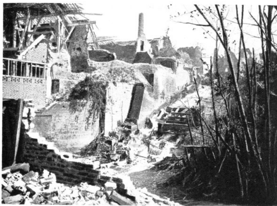
RUINED WORKS ON RIVER ANCRE, AND CASCADE.
