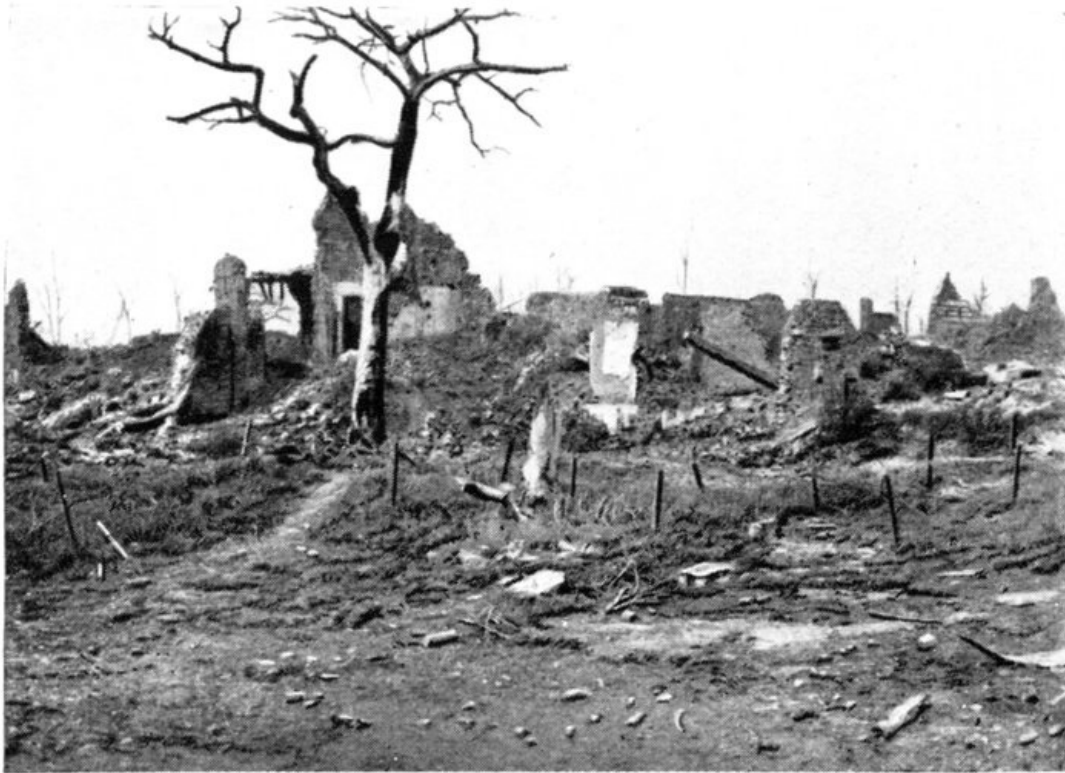
MONT-ST.-QUENTIN. RUINED HOUSES.
