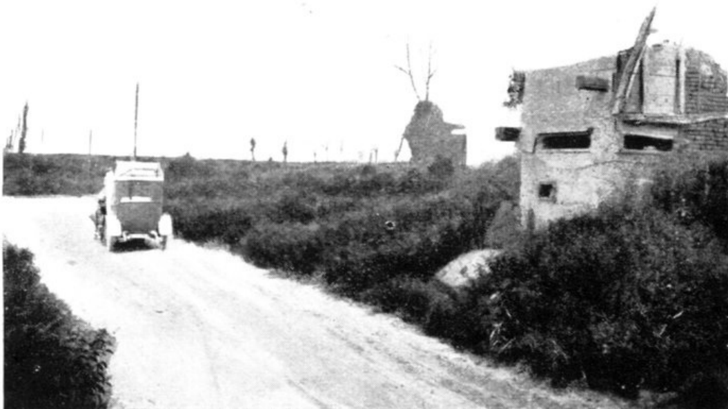
ON LEAVING HERBÉCOURT—GERMAN BLOCKHOUSE AT THE CORNER OF THE ROADS TO CAPPY ( on the right ) AND DOMPIERRE ( on the left ).
