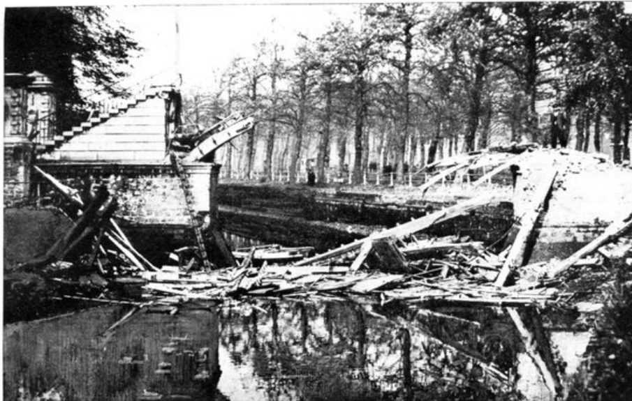
NAPOLÉON BRIDGE DESTROYED BY THE RETREATING GERMANS (see p. 52)
