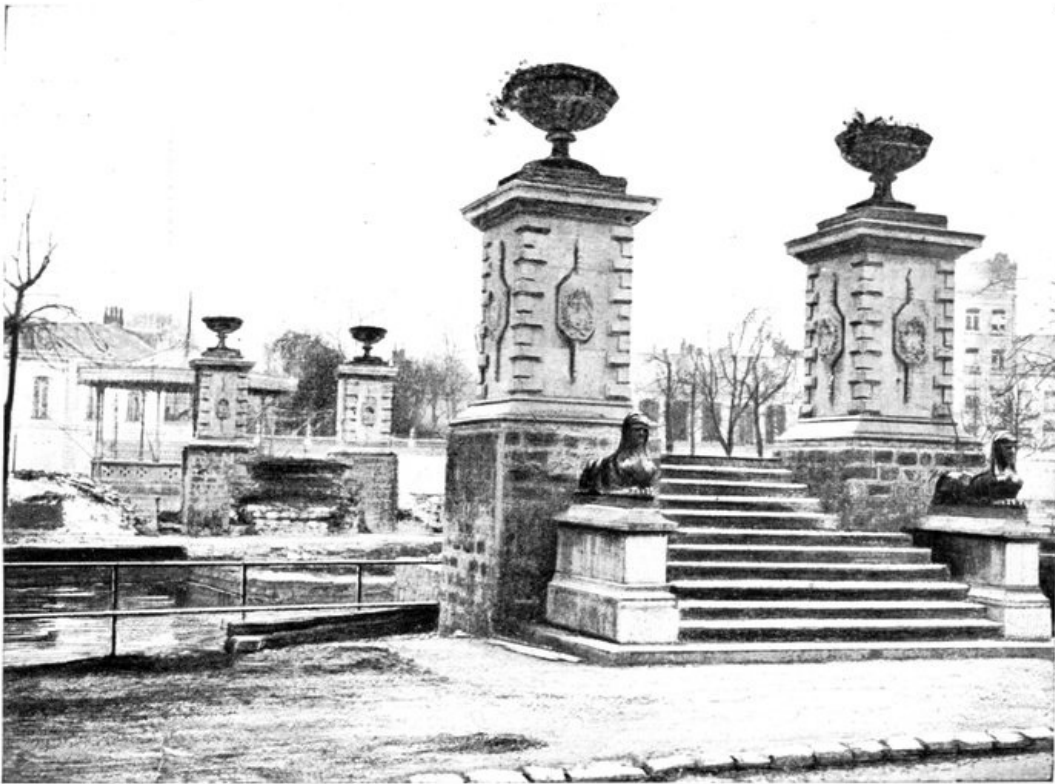
NAPOLÉON BRIDGE (January, 1919).
