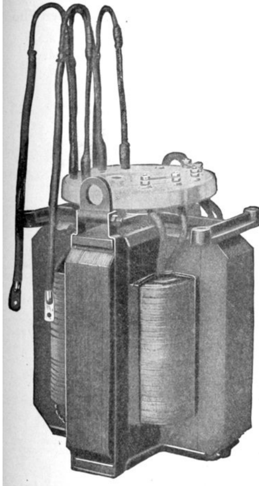
FIG. 1,944.—General Electric 10 kva., (type H) transformer removed from tank. That part of the steel core composing the magnetic circuit outside of the winding is divided into four equal sections. Each section is located a sufficient distance from the winding so that all portions of the winding and core are equally exposed to the cooling action of the oil. On all except the very smallest sizes the winding is divided by channels and ducts through which a continual circulation of oil is maintained. The result is uniform temperature throughout the transformer, thus eliminating the detrimental effects of unequal expansion in the coils with consequent rubbing and abrasion of the insulation.
