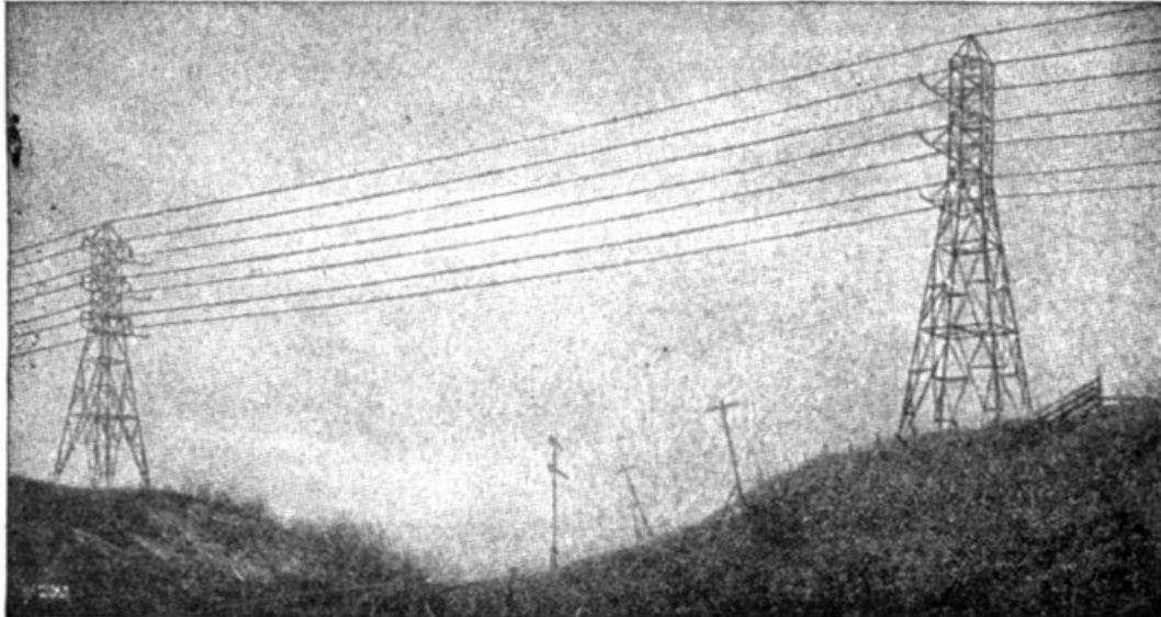
FIG. 2,193.—Line of the Schenectady Power Company crossing the tracks of the Boston and Maine Railroad near Schaghticoke.
