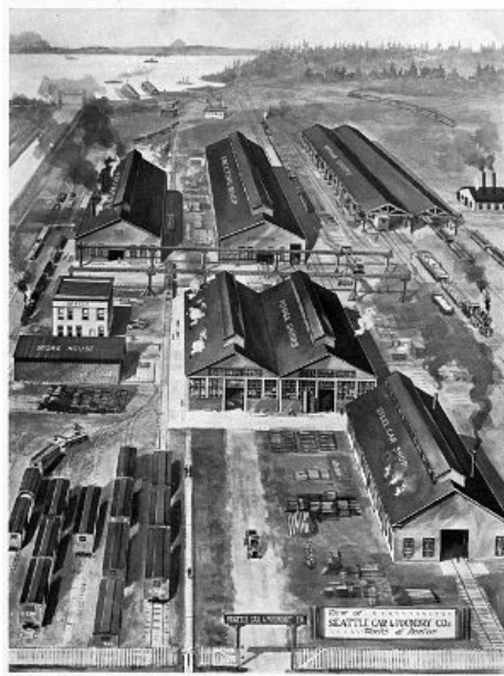
WORKS AT RENTON, WASH.
