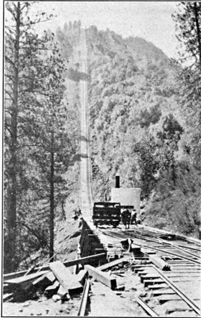
Yosemite Valley Lumber Co., Merced, Cal., logging operations. This incline is 8700 feet long, part of which is 80% grade. Equipped by Seattle Car and Foundry Company. For detailed description of equipment see Yosemite Grade Destroyer.
