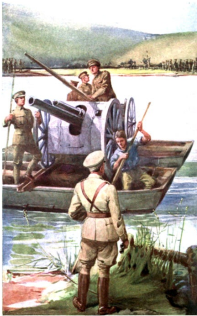
Royal Engineers at Pontooning Work.
