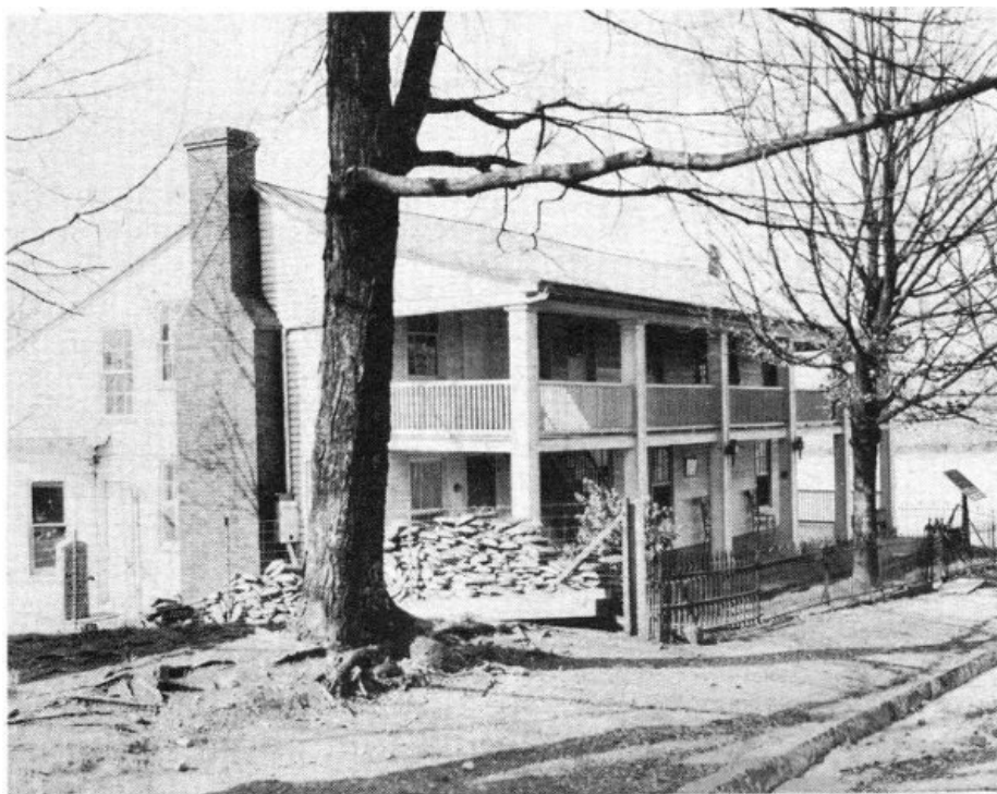
Dover Tavern, General Buckner's headquarters and scene
