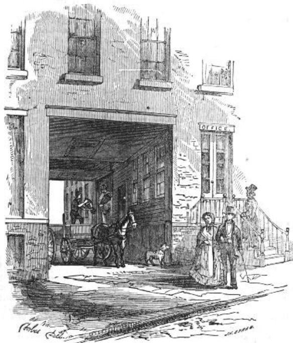
GATEWAY ENTRANCE TO BOARDMAN & GRAY'S FACTORY.
