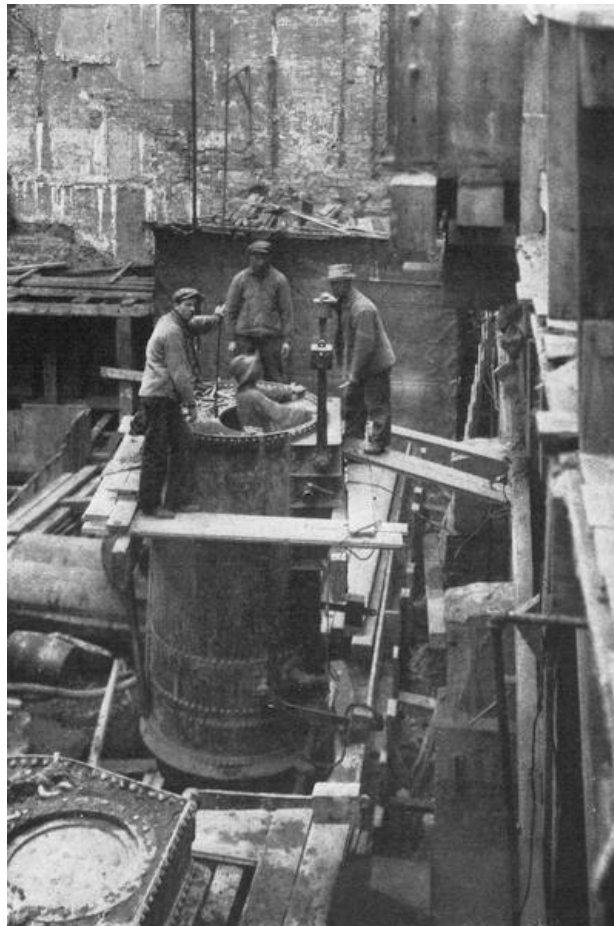
THE AIR-LOCK OF A PNEUMATIC CAISSON
