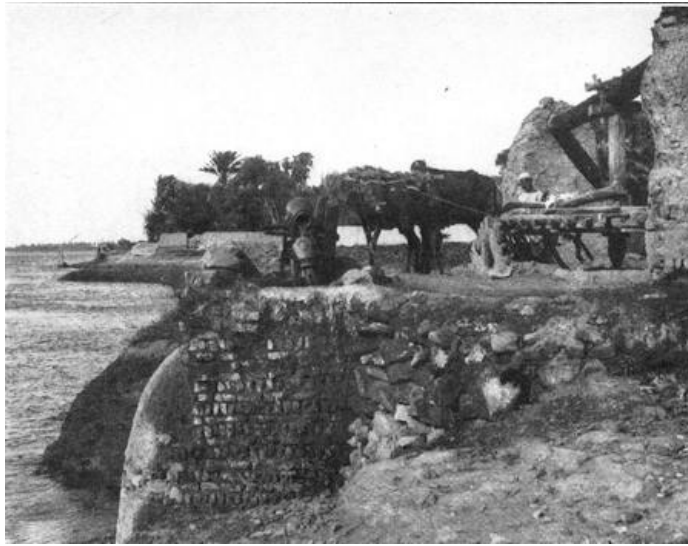
RAISING WATER WITH A CHAIN OF POTS A primitive pump still used in Egypt
