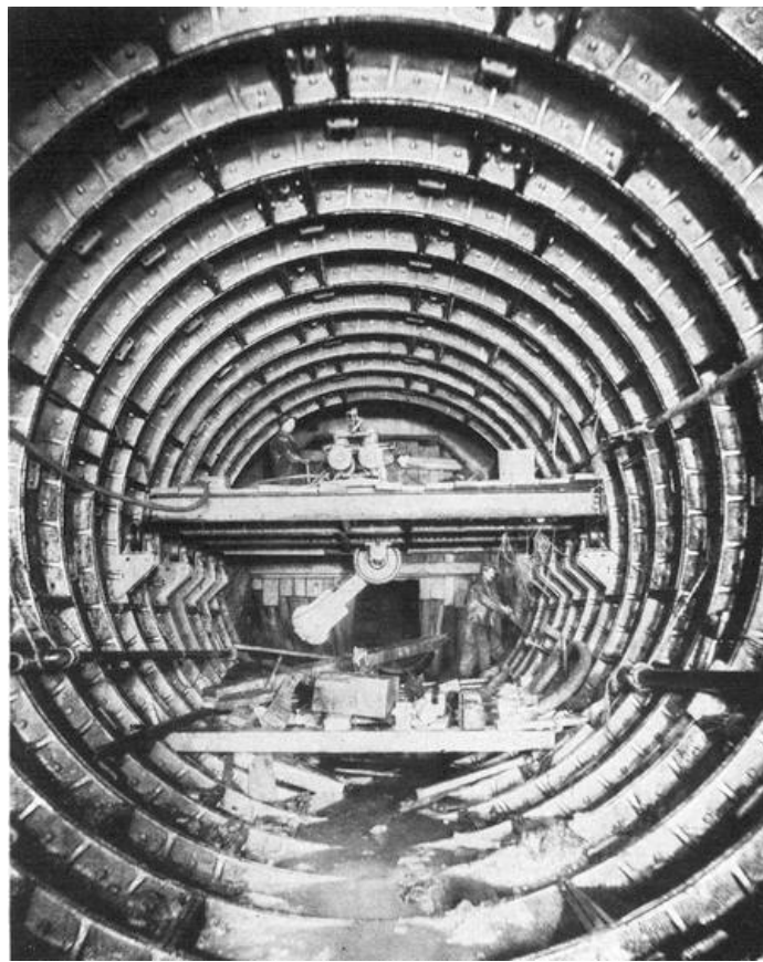
SUBAQUEOUS TUNNEL, SHOWING THE SHIELD IN THE BACKGROUND
