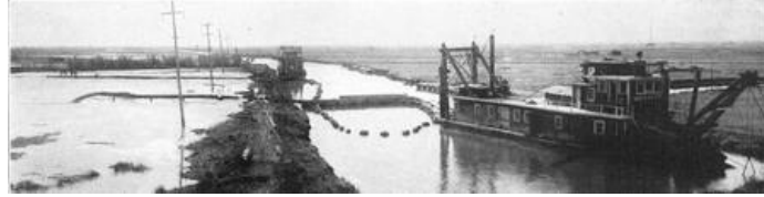
A SUCTION DREDGE EXCAVATING A CHANNEL AND BUILDING NEW LAND
