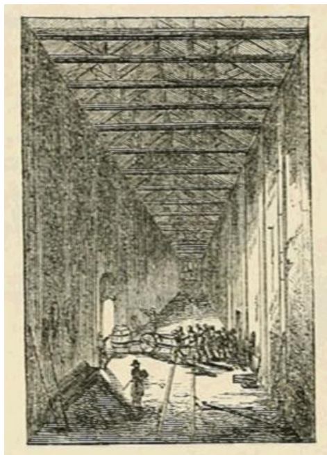
PLATE GLASS CASTING. BRINGING OUT THE POT.
