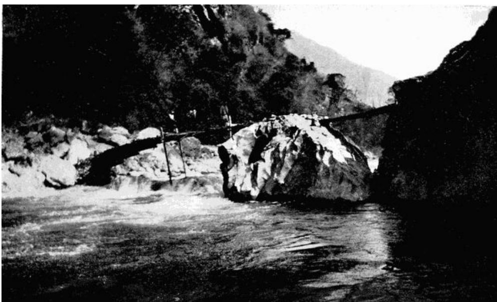
RUSTIC BRIDGE CROSSING LITANG RIVER ON THE ROAD TO MULI.
