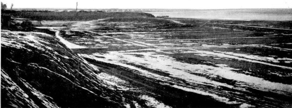
SOUTH BANK OF YELLOW RIVER, WITH VIEW OF RAILWAY BRIDGE.
