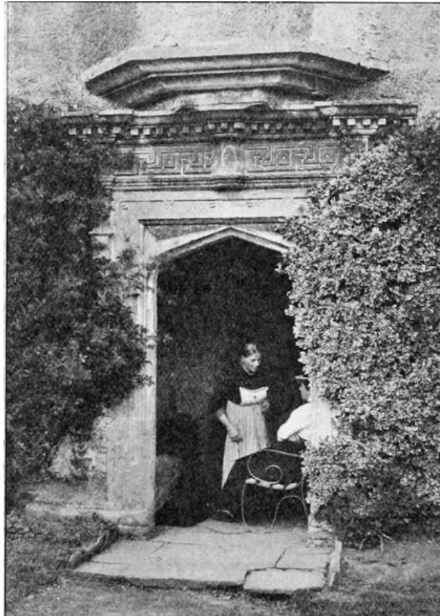
65.—DOORWAY AT NAILSEA COURT, SOMERSET.
