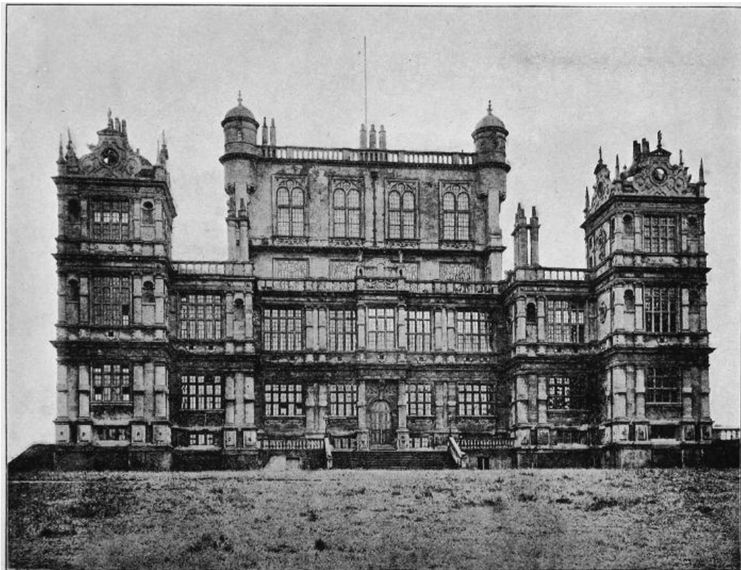
WOLLATON HALL, NOTTINGHAMSHIRE.
