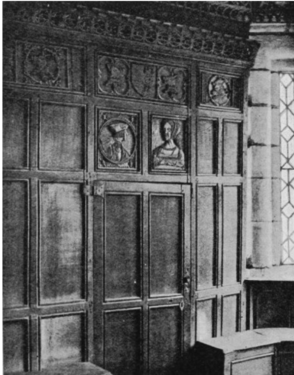
HADDON HALL, DERBYSHIRE. A SIDE OF THE BAY- WINDOW IN THE DINING-ROOM (1545).
