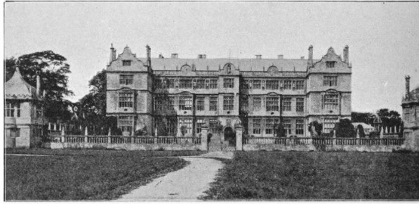
48.—MONTACUTE HOUSE, SOMERSET. WEST FRONT, WITH COURT AND GARDEN-HOUSES (1580).
