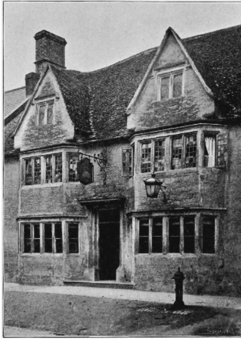
191.—THE "SWAN" INN, LECHLADE, GLOUCESTERSHIRE.
