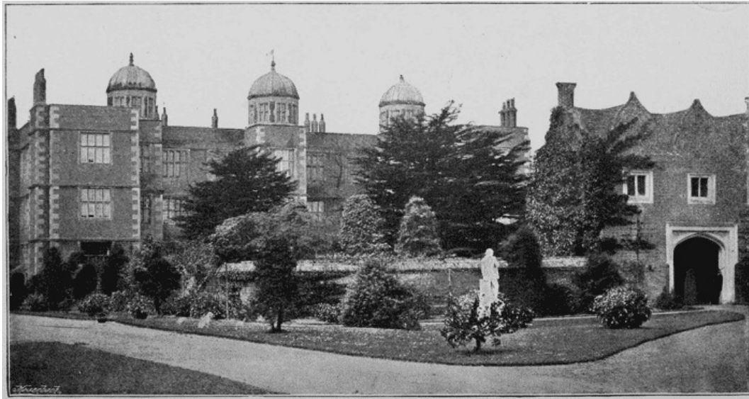
DODDINGTON HALL, LINCOLNSHIRE. ENTRANCE FRONT WITH GATEHOUSE (1595).
