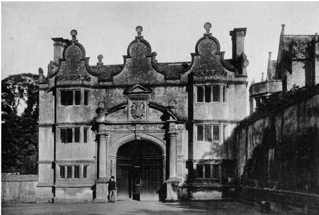
STANWAY, GLOUCESTERSHIRE (ABOUT 1630). THE GATEHOUSE.
