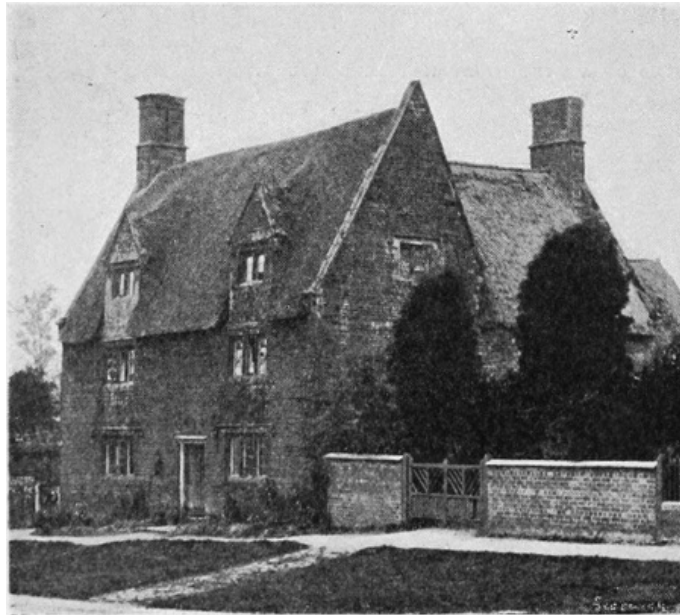
100.—A NORTHAMPTONSHIRE COTTAGE.
