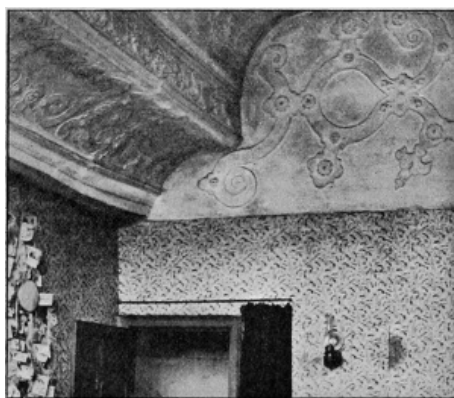
163.—COVED CEILING, BECKINGTON ABBEY, SOMERSET.
