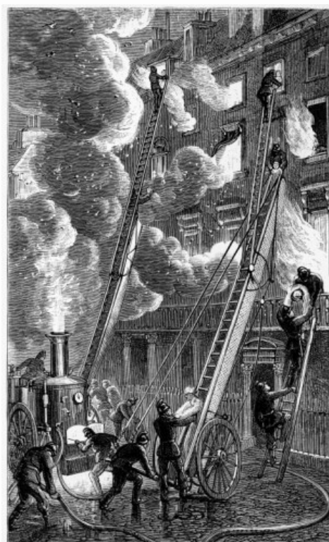
FIRE-ESCAPE AND STEAM FIRE-ENGINE IN ACTION (From a drawing supplied by the Royal Society for the Protection of Life from Fire)
