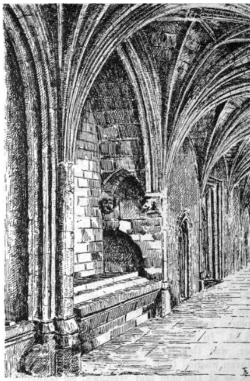
Fig. 8. Worcester: lavatory in west walk of cloister.
