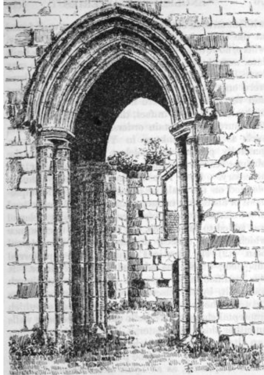
Fig. 5. Mount Grace priory: tower-arches and nave from N.E.
