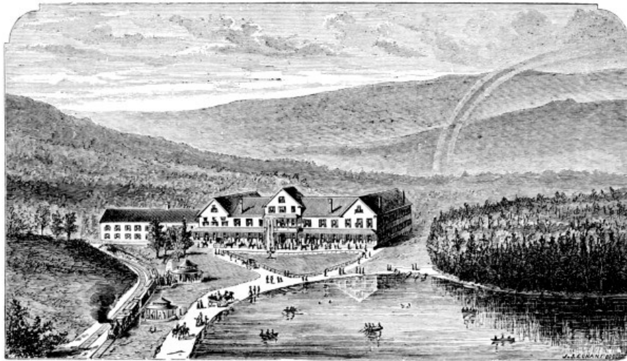
CRAWFORD HOUSE, WHITE MOUNTAIN NOTCH.
