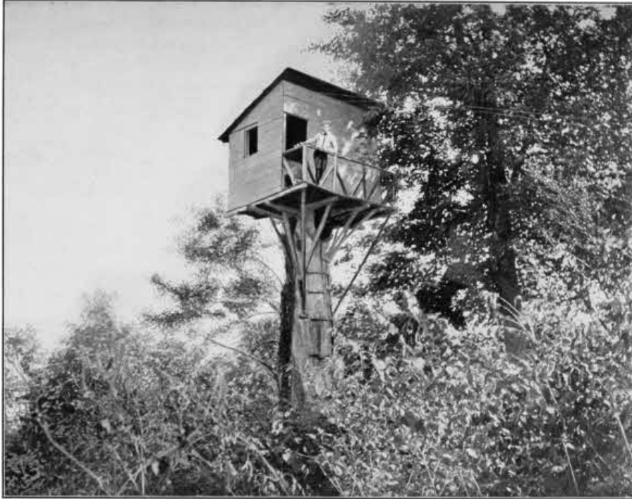
Tree-top House. 6 × 10 feet, 35 feet from ground to floor.
