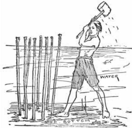
FIG. 84.—Using a Home-made Maul.
