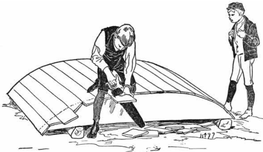
FIG. 29.—The Ends may be Sawed off Flush.
