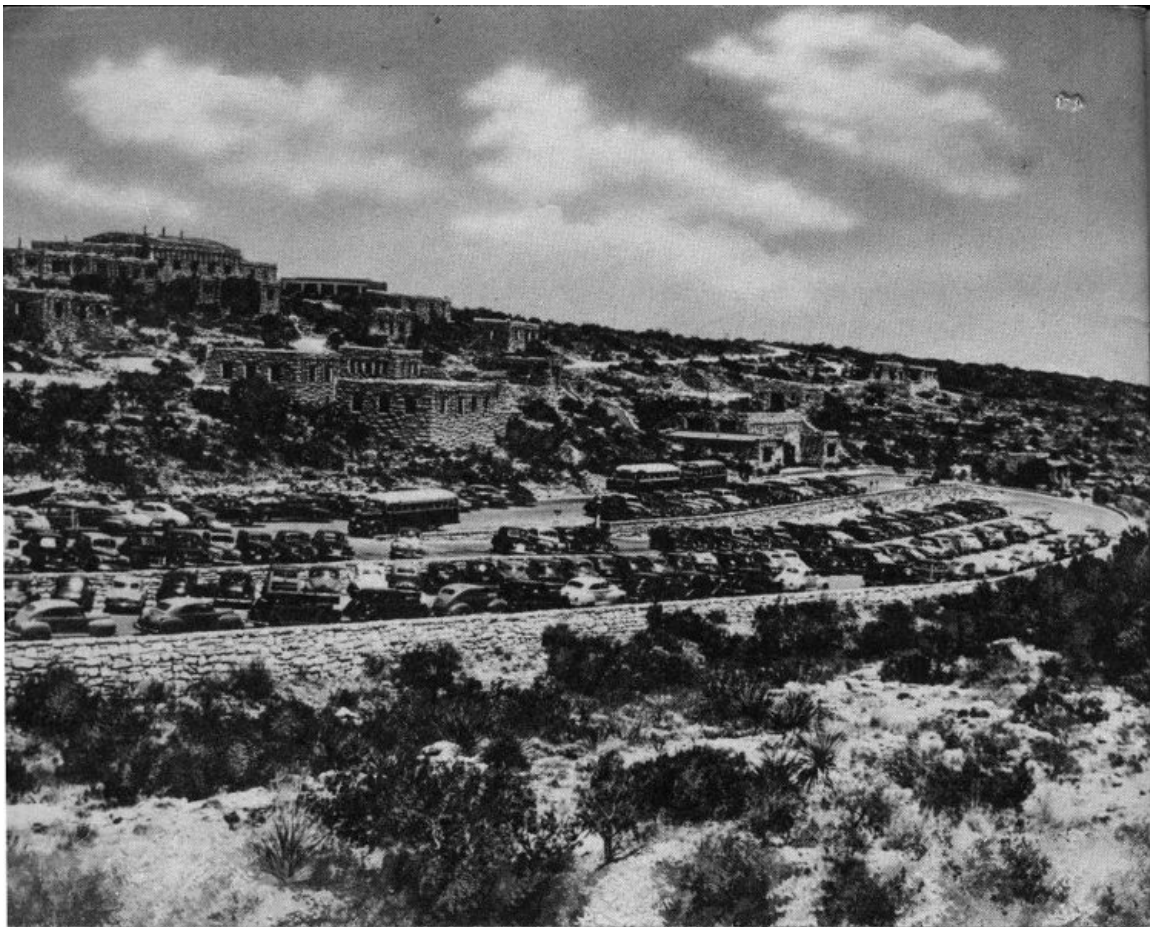
Government Buildings and Parking Terraces Adjacent to the Entrance to Caverns
