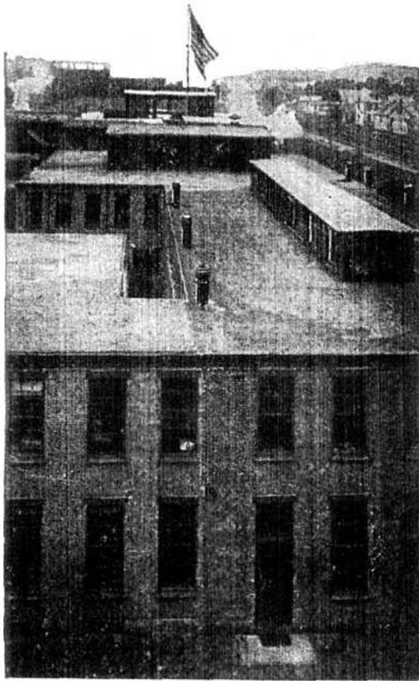
FIGS. 2,739 and 2,740.—Substituting mechanical draught in place of chimney. The relative proportions of a brick chimney, and of the smoke pipe required when mechanical draft is introduced are forcibly shown in the illustrations, which show the works of the B.F. Sturtevant Co., at Jamaica Plain, Mass. The removal of the boilers to a position too far distant from the existing chimney to permit of its longer fulfilling its office, led to the substitution of an induced draft fan and the subsequent removal of the chimney. The present stack or smoke pipe, barely visible in fig. 2,740, extends only 31 feet above the ground, and no trouble is experienced from smoke.
