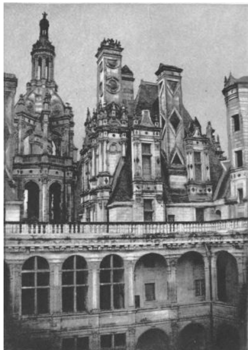
Portion of the Roof of the Château of Chambord
