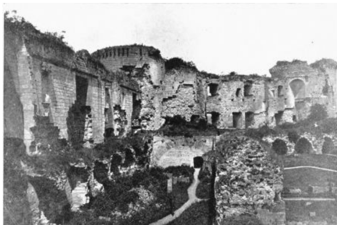
COUCY—INTERIOR, SHOWING THICKNESS OF WALLS.
