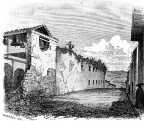
WHAT THE EARTHQUAKES LEFT
