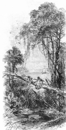
ANTICS ON THE BRIDGE.
