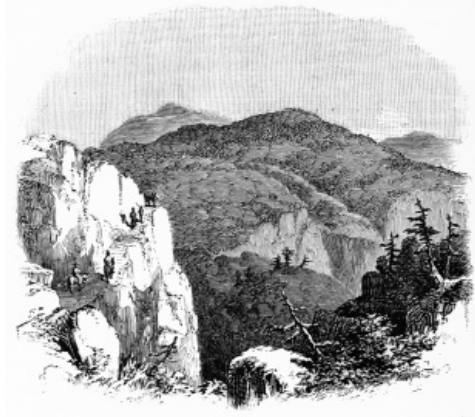
ROAD CUT IN THE ROCKS.
