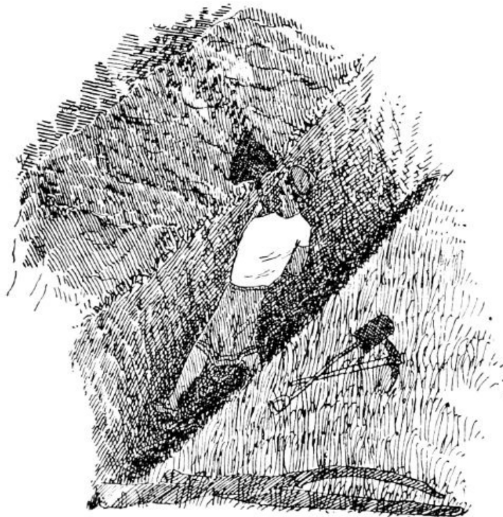
Digging Ye First Corral Ditch.
