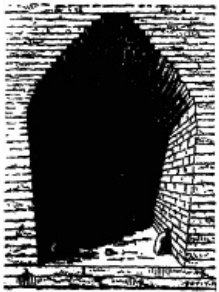
Fig. 4.—Corbelled vaulting at Mugheir (after Taylor).
