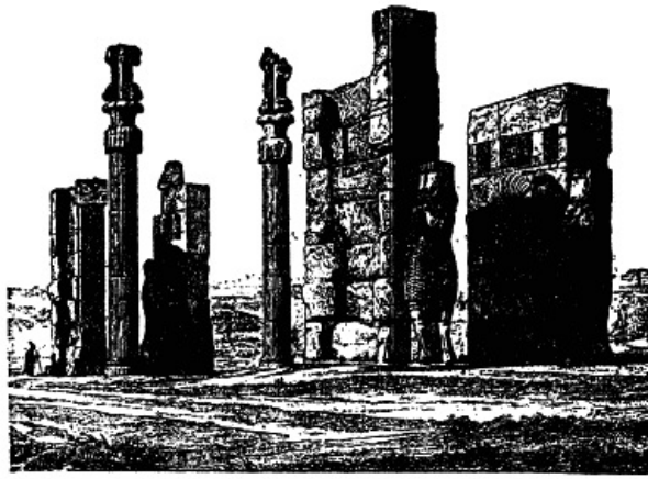
Fig. 134.—Portico at Persepolis (after Flandin and Coste).
