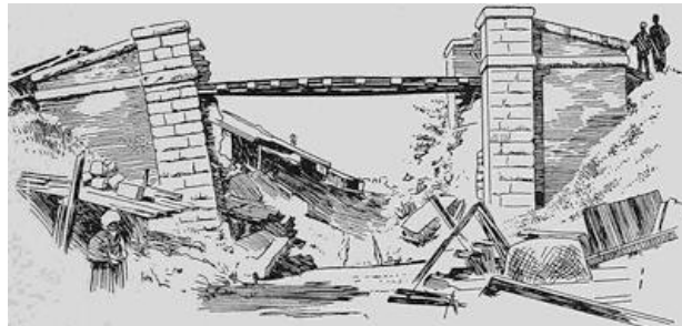
FIG. 65.—The Biwajima railroad bridge in Japan after the earthquake of 1891 (after Milne and Burton).
