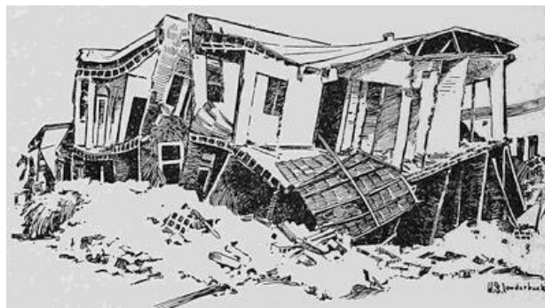
FIG. 85.—House wrecked in San Francisco earthquake of 1906 because the floors and partitions were not securely fastened to the walls (after R. L. Humphrey).
