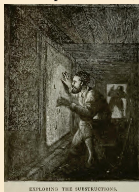
EXPLORING THE SUBSTRUCTIONS.
