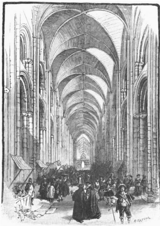
INTERIOR OF OLD ST. PAUL'S.
