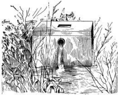
FIG. 126.—Concrete cover for a spring.
