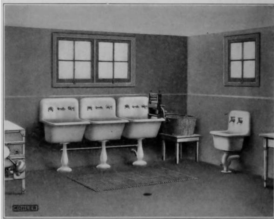
FIG. 83.—Enamel wash trays in a basement laundry.
