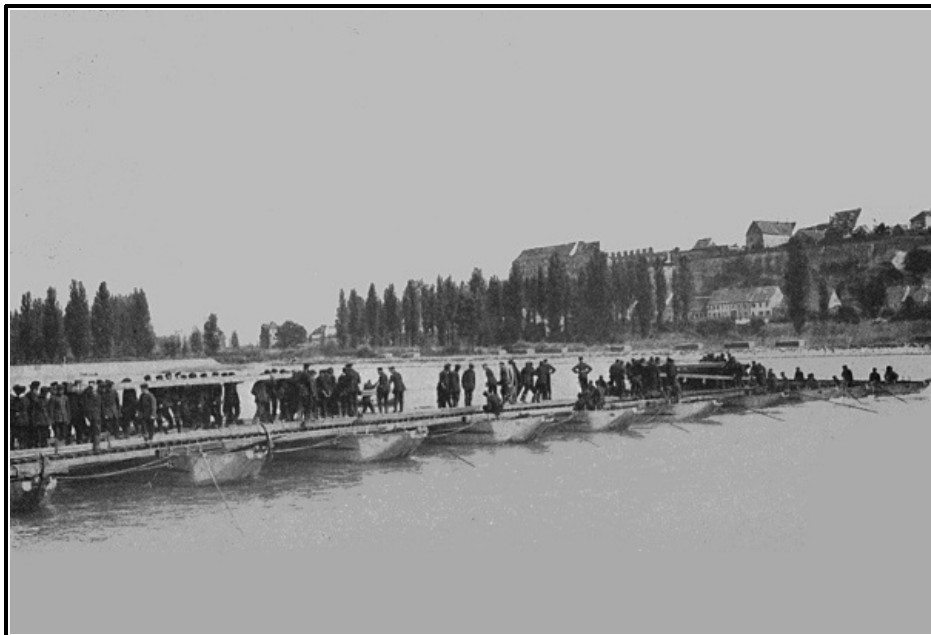
Building a Pontoon Bridge
