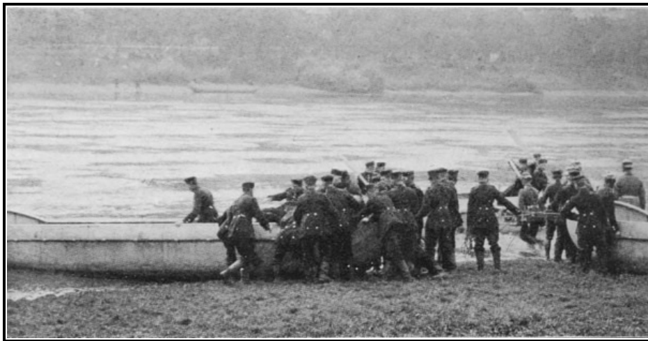
Floating the pontoons
