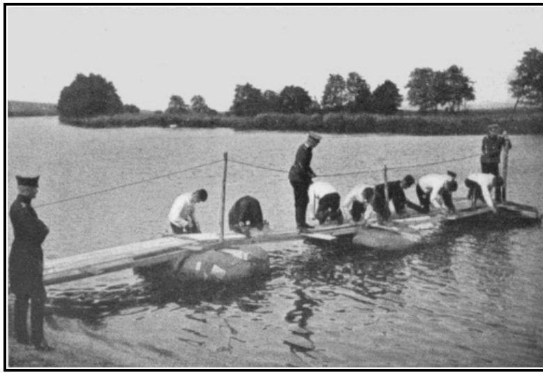
Building a Bridge with Sacks
