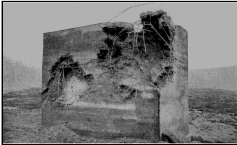
Effect of Two Shells on a Six-Foot Reinforced Concrete Wall
