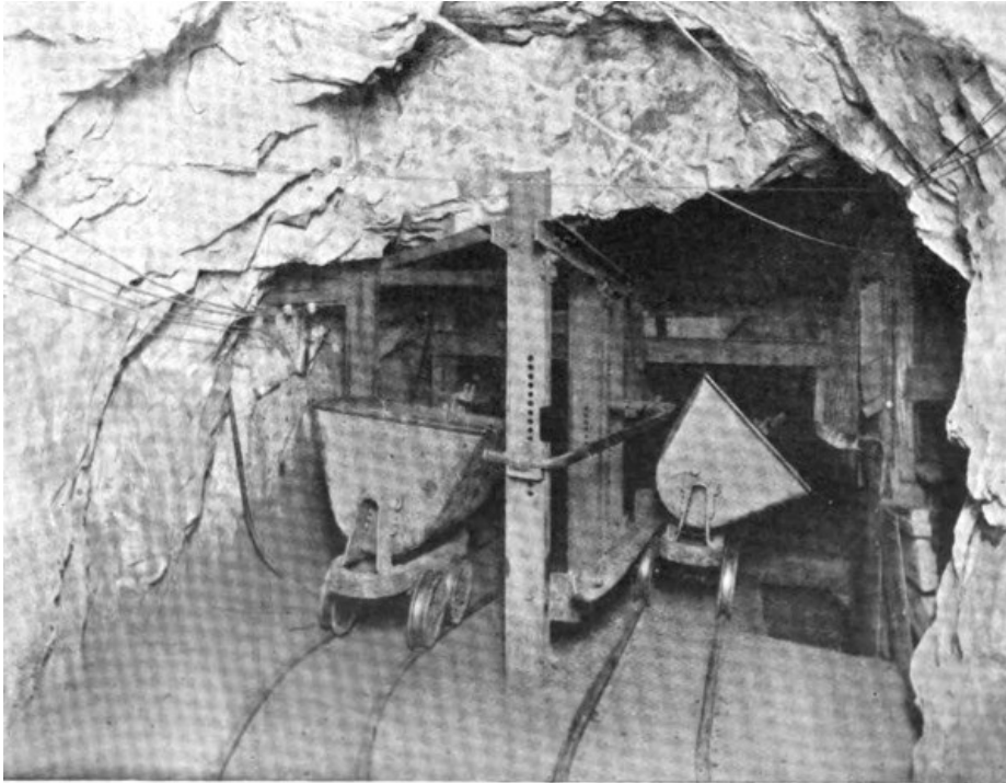
THE FIVE HUNDRED FEET LEVEL OF THE WESSELTON MINE, SHOWING AUTOMATIC TIPS AND TRUCK TIPPING INTO THE CHUTE INTO WHICH WOOD WAS THROWN.
