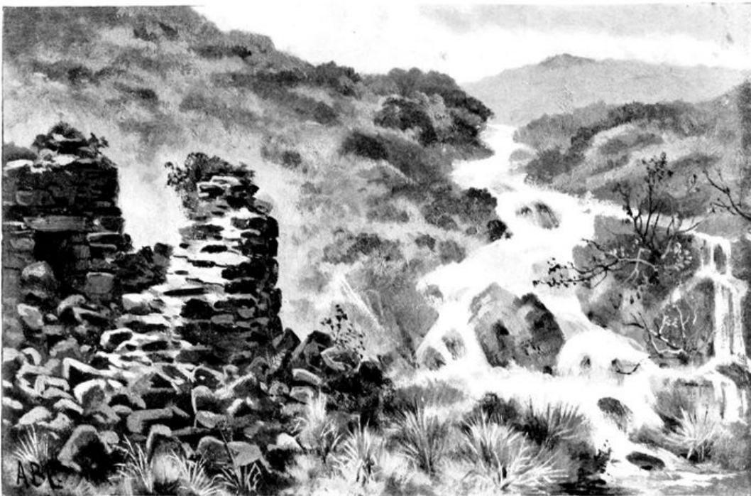
BLOWING-HOUSE UNDER BLACK TOR
