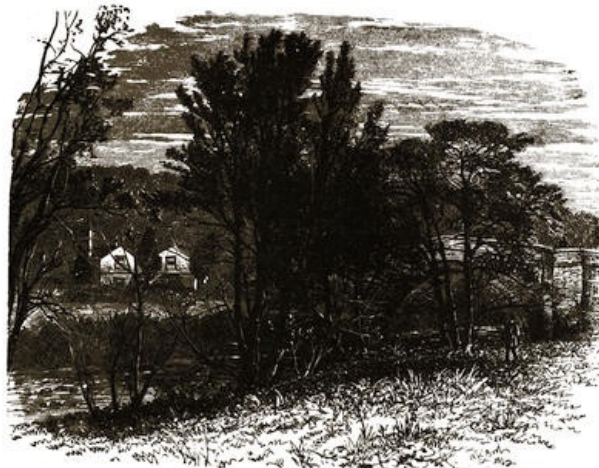
Edensor Mill Lodge and Beeley Bridge.
