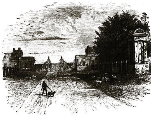
The Grand Entrance-Lodge at Baslow.
