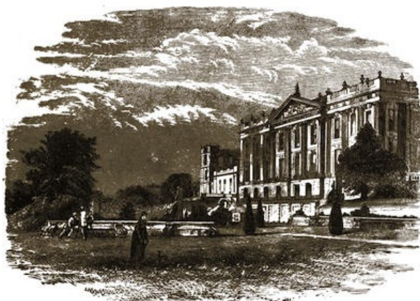
West Front from the South.
