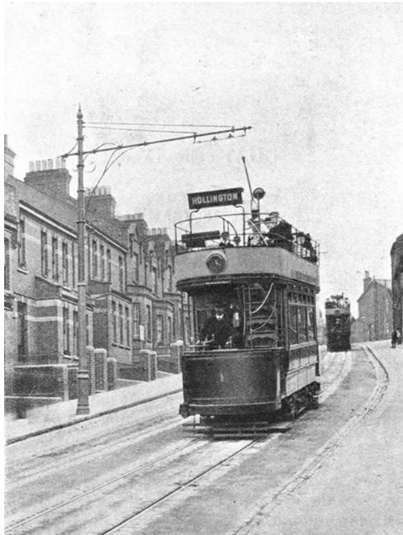
Fig. 2. A typical electric tramway on the overhead system.—The trolley standard carries the wires for supplying current to the cars on both the up and down tracks. The driver has his left hand on the controller handle and his right hand on the brake handle. (Photograph reproduced by courtesy of Dick, Kerr and Company, Limited.)
