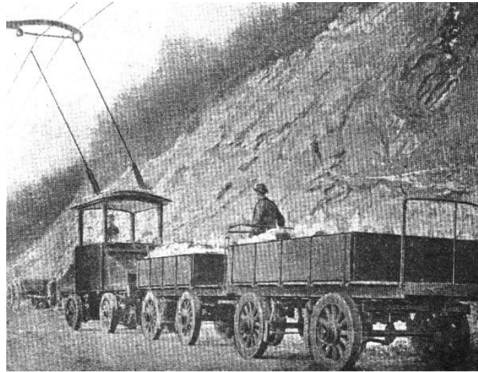
Fig. 7. The 'auto-trolley' system of electric traction applied to the haulage of goods in a German quarry. (From Electrical Industries .)
