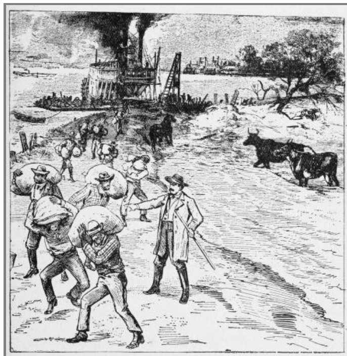
STRUGGLE TO HOLD THE LEVEE.
