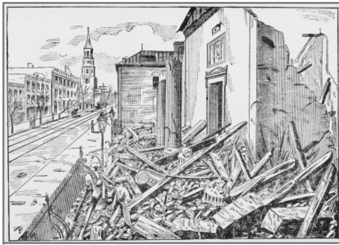
WRECK OF THE CHARLESTON EARTHQUAKE.
