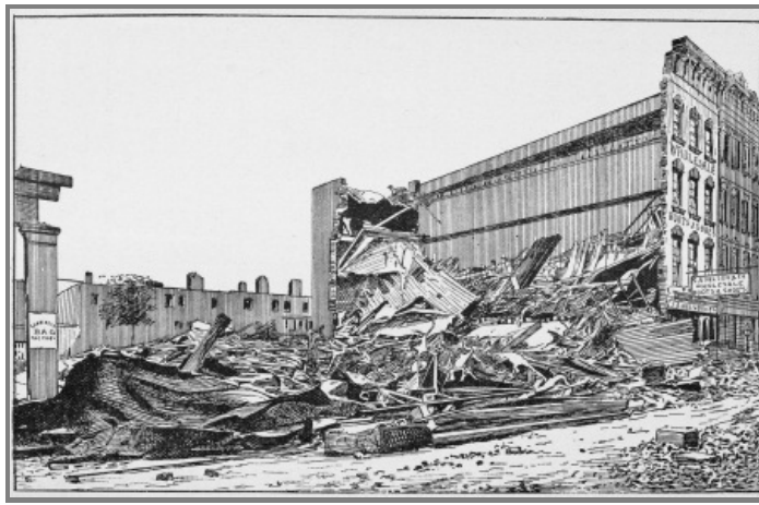
WRECK OF FACTORY, CHARLESTON.
