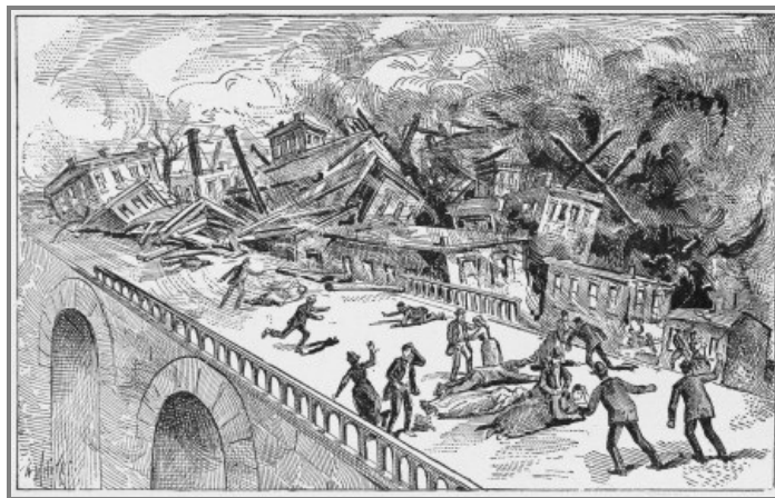
AT THE STONE BRIDGE.
