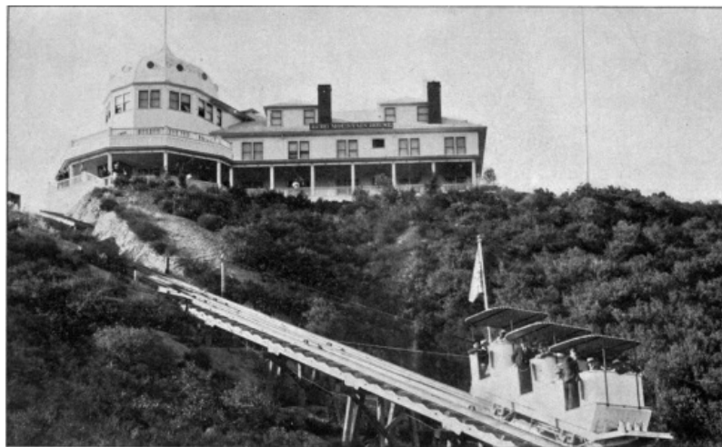
ECHO MOUNTAIN HOUSE AND CAR ON THE 48 PER CENT. GRADE, MT. LOWE RAILWAY.
