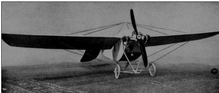
THE NIEUPORT MONOPLANE Self-Starting with an 18 hp. motor (From The Air Scout )
