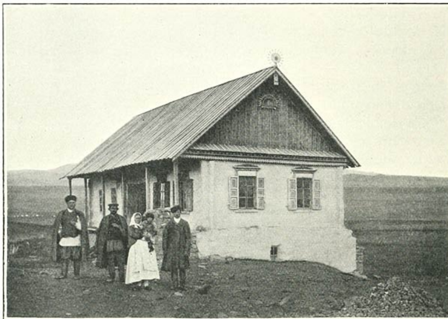
FIG. 100. HOUSE AT NOVO-MICHAELOVKA.
