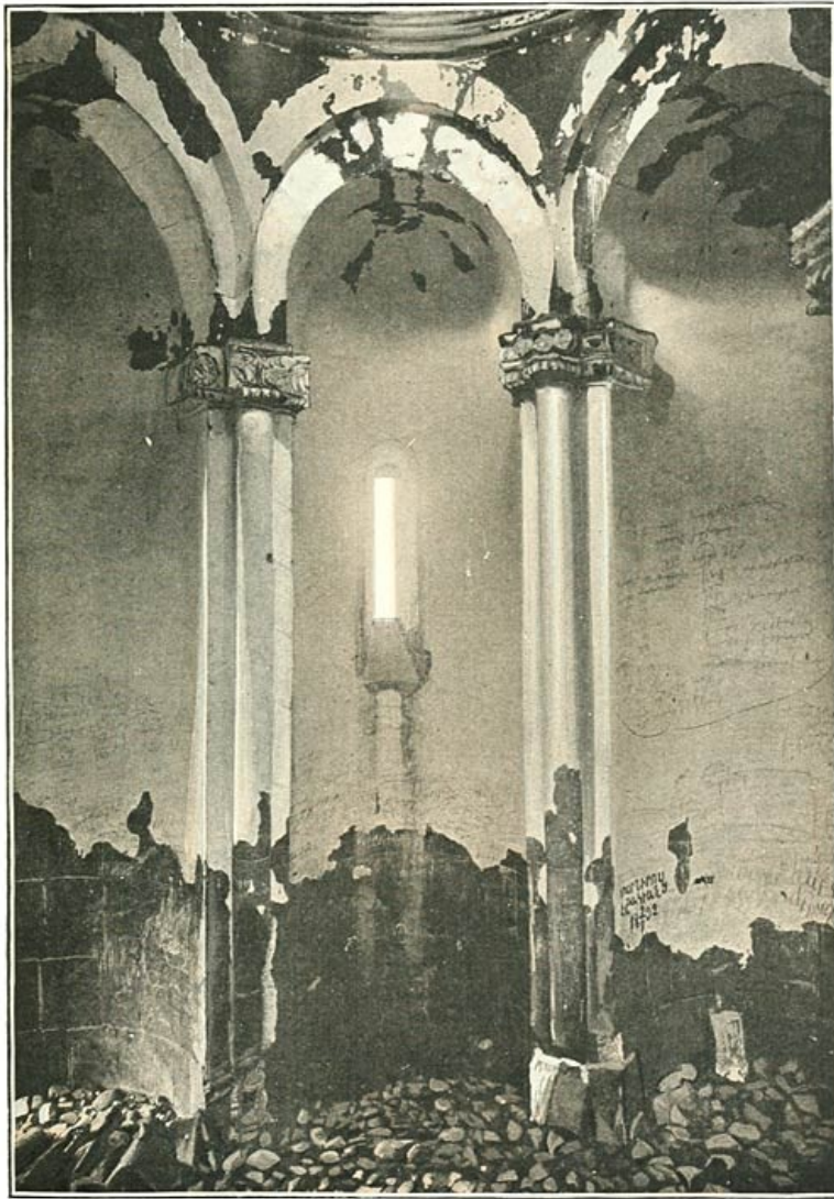
FIG. 87. ANI: INTERIOR OF THE CHAPEL OF ST. GREGORY.
