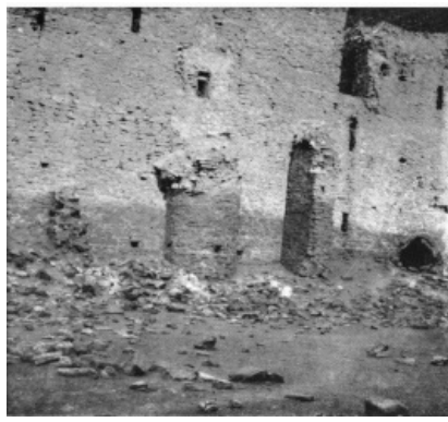
FIG. 1. Ukhaiḍir, remains of stair.
