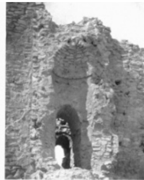
FIG. 2. Ukhaiḍir, detail of tower chamber.
