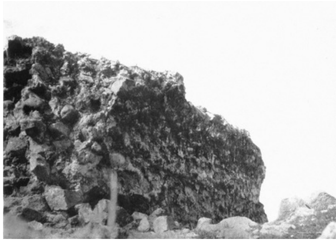
FIG. 2. Palace of Khusrau, vault of room 71.
