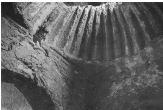
FIG. 2. Ukhaiḍir, room 4, south-west portion of dome.
