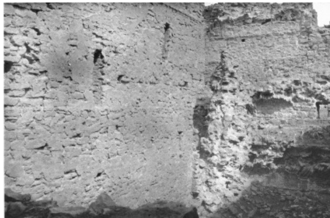
FIG. 1. Ukhaiḍir, north-east angle of court A.
