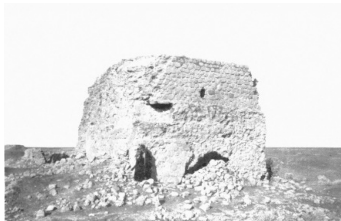
FIG. 3. Qṣair, exterior from south.
