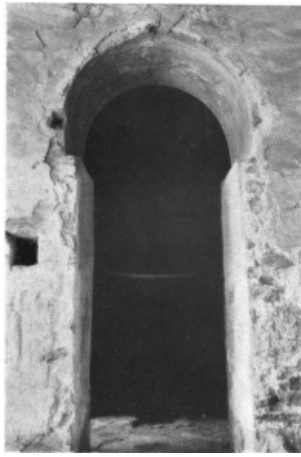
FIG. 1. Ukhaiḍir, door between rooms 44 and 45 from room 44.
