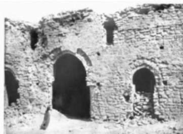
FIG. 4. Ukhaïdir, court c, eastern half of north façade.
