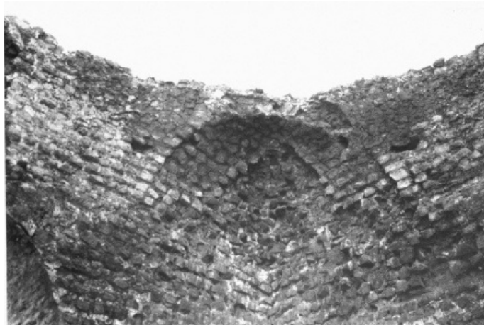
FIG. 2. Chehâr Qapû, hall 54, squinch in south-west corner.
