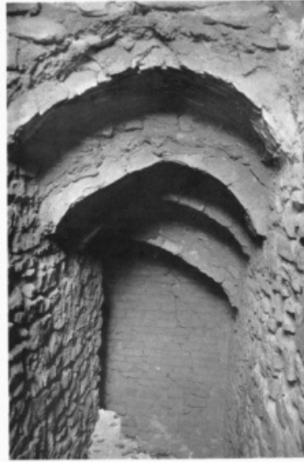
FIG. 2. Ukhaiḍir, vault of south-west stair out of great hall.
