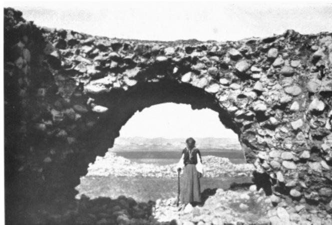
FIG. 2. Palace of Khusrau, gateway between courts u and v, west arch.
