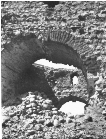
FIG. 1. Chehâr Qapû, hall 54, exterior of south door.
