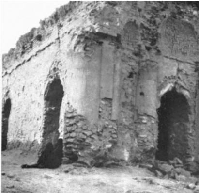
FIG. 1. Ukhaiḍir, room 29 and south side of central court.
