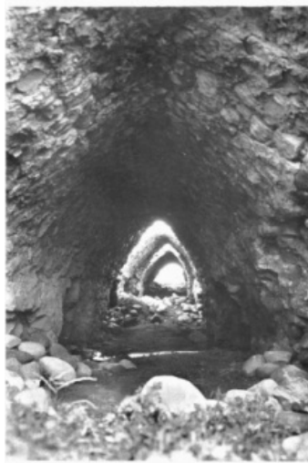
FIG. 1. Palace of Khusrau, corridor 103, east side.
