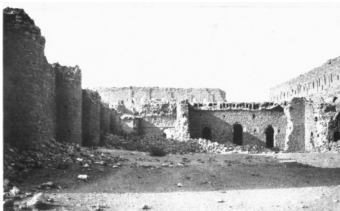
FIG. 2. Ukhaiḍir, east annex, from south.
