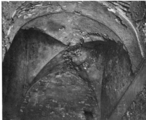
FIG. 2. Ukhaïdir, groin in north-east angle of corridor 28.
