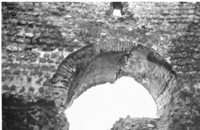
FIG. 2. Chehâr Qapû, hall 54, interior of south door.
