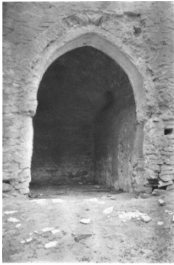
FIG. 1. Ukhaidir, south door of room 44.
