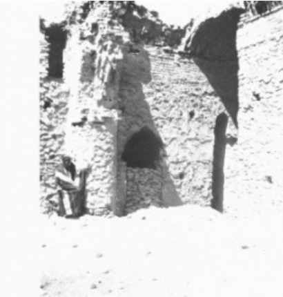
FIG. 3. Ukhaiḍir, south-west angle of passage 36.
