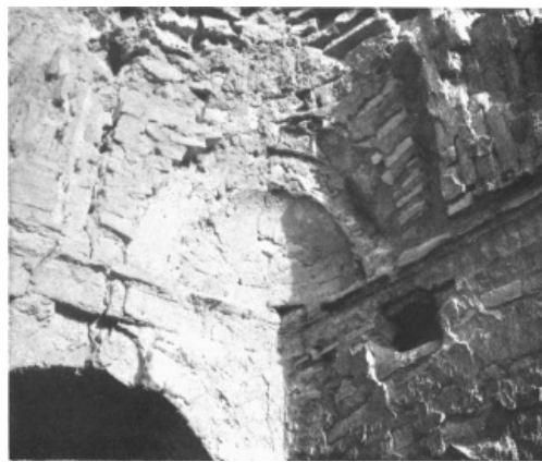
FIG. 2. Ukhaiḍir, squinch in north-west angle of gallery 134.
