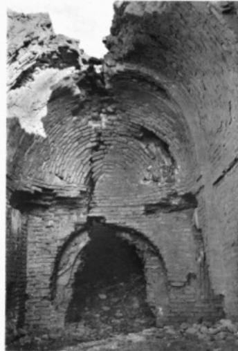
FIG. 2. 'Atshân, west door of room 6, from west.
