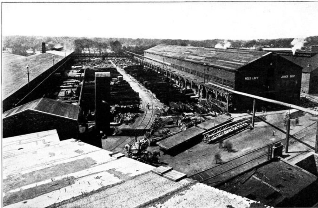
VIEW IN THE GROUNDS OF THE FORE RIVER SHIPBUILDING COMPANY, QUINCY, MASS.
