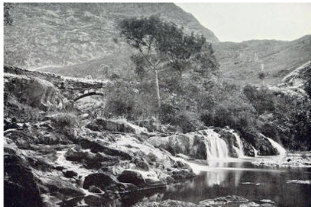
NANT BRIDGE, CARNARVON
