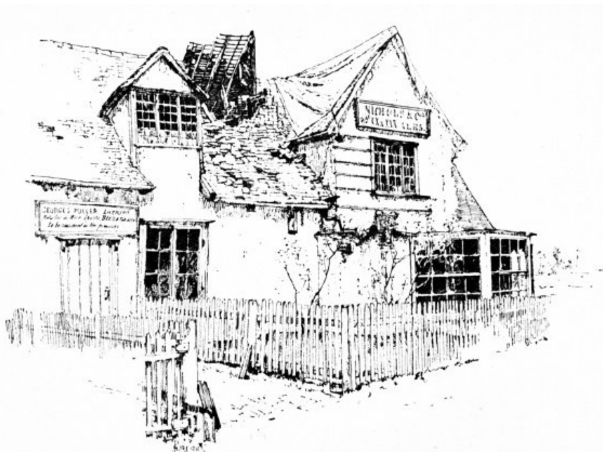
ROSE INN AT PELDON (after the earthquake).
