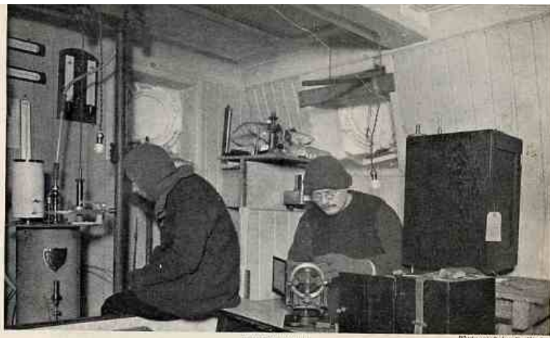
THE ROOKERY Photograph by F. Hurley The scientific laboratory with Hussey examining the Binn's anemometer and James removing rime from the electro- The electrograph is on the Hussey James
